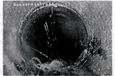
Illustration 3: Slipped joint, infiltration
