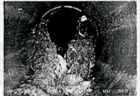
Illustration 6: Slipped joint, root ingress
