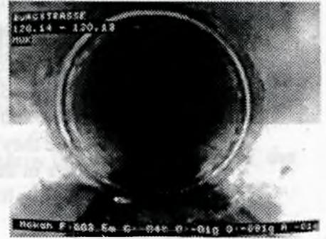
Illustration 15: Slipped joint + longitudinal cracks
