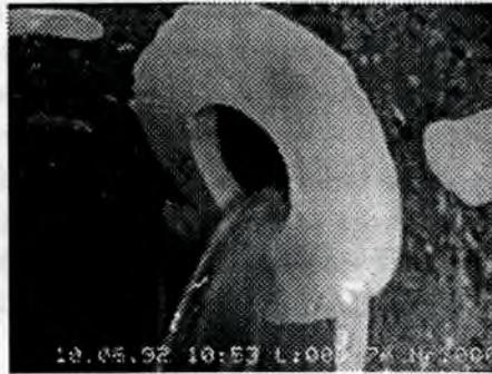
Illustration 14: Broken out lateral with cracking
