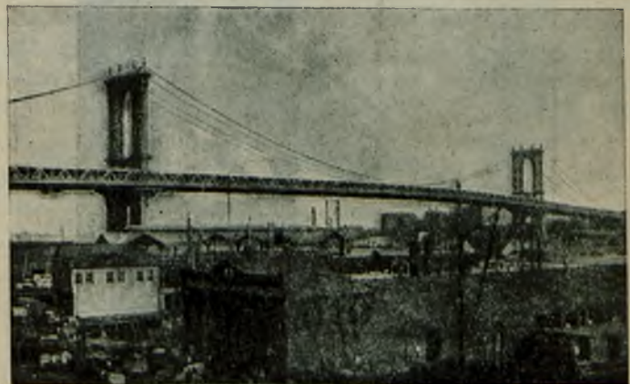
Rys. 10. Manhattan Bridge, New York.
