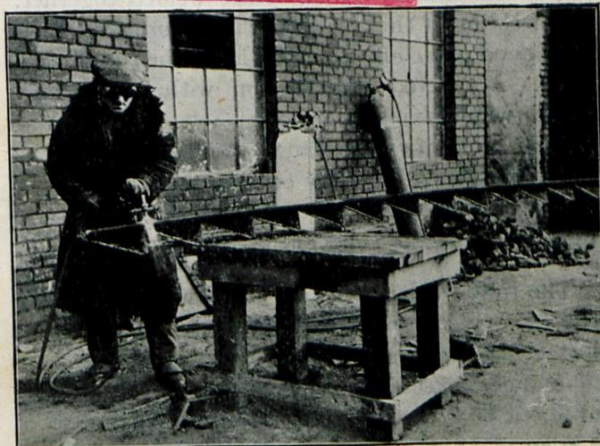
Fig. 3. — Cutting I-beams into small triangles.
