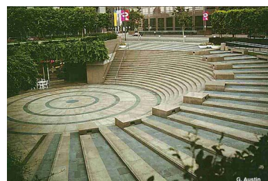
151. Schody w krąg. Museum of Contemporary Art , Los Angeles, 1983–87, POD, Inc., Landscape Architects
