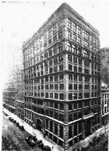
9. Arch. W. L. B. Jenney. „Home-Insurance-Building“ w Chicago. R. 1885.
