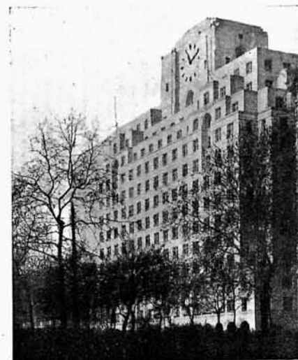
Arch. M. Joseph. Gmach T-wa Shell w Londynie. (The Architectural Review).
