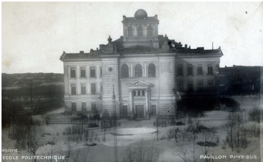
Fig. 5. The Physics Building in its final stage of construction
