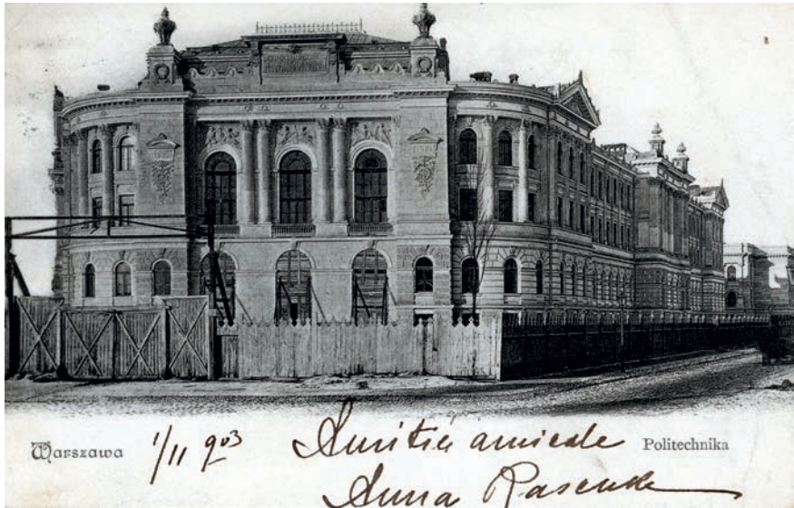
Fig. 4. The Main Building at the final stage of construction in 1901. – View from former Wiejska Street
