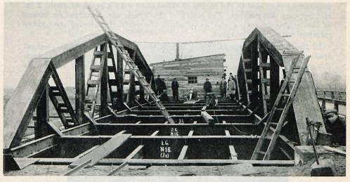
FIG. 4-WELDED HIGHWAY BRIDGE IN POLAND NEARING COMPLETION
