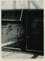
FIG. 3—WELDED CONNECTION BE-TWEEN STRINGER AND FLOORBEAM Adoption of this type of connection permitted calculation of the stringers as continuous beams and resulted in a saving of about 12 per cent of steel in the crossbeams
