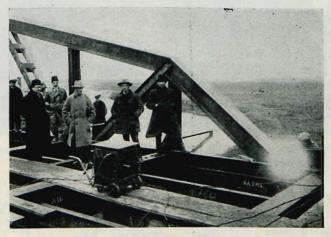
FIG. 2--WELDING AN END POST ON THE POLISH HIGHWAY BRIDGE Note the welding generator in the foreground
